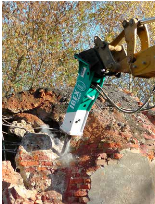
BREAKING OF MASONRY
