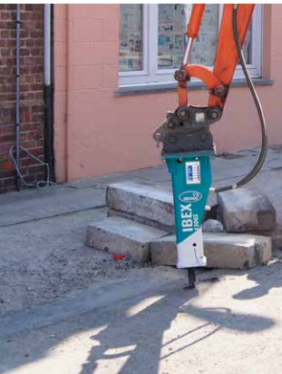
ASPHALT AND PAVING
