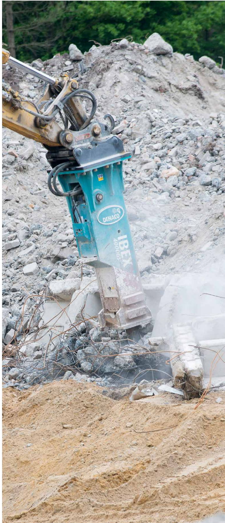
BREAKING OF MASONRY
