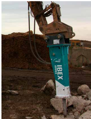
DEMOLITION OF BUILDINGS
