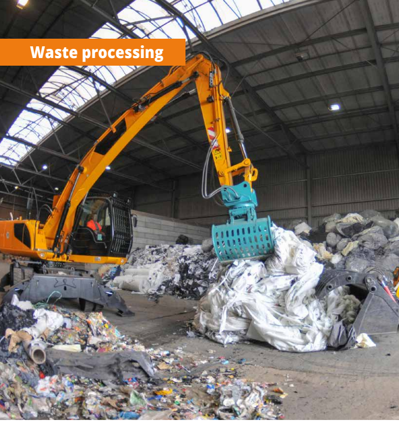
Moving construction materials
