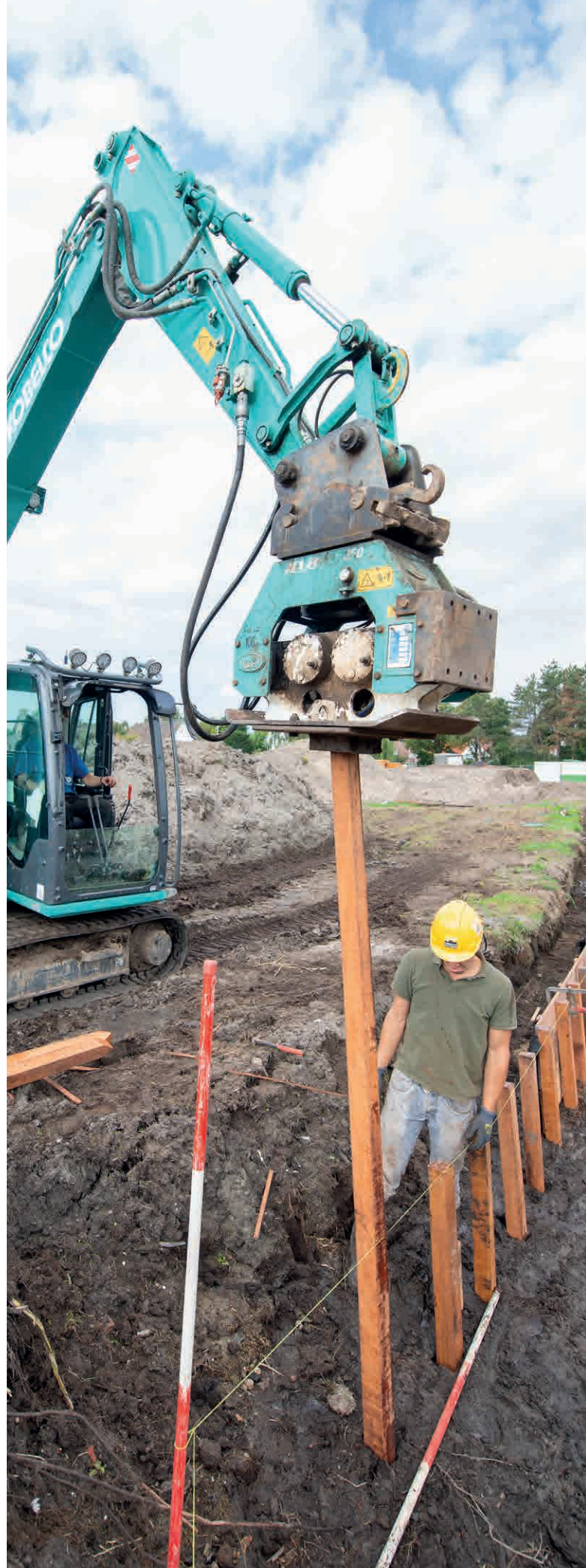
Driving of sheet piles
